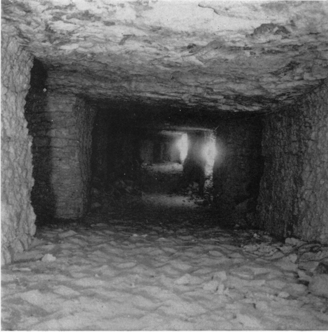
1. The main gallery half filled with sand
